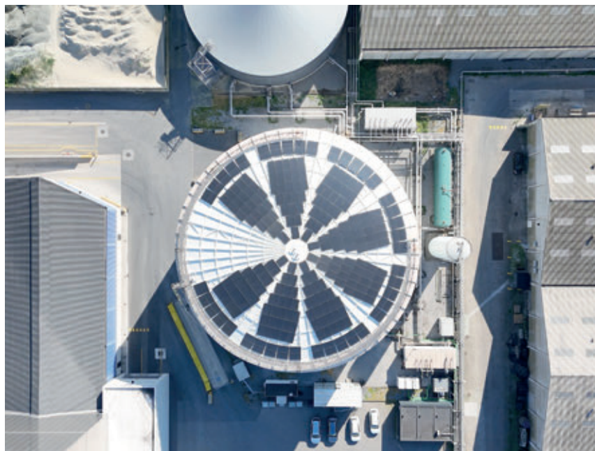
Fertigent installed solar panels on the roof and on the sun-facing sides of the tank walls.
