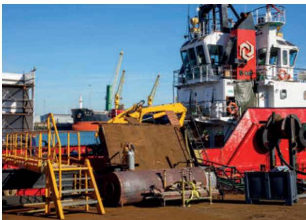
The yard has also built an extension to provide vehicular access to the dock.
