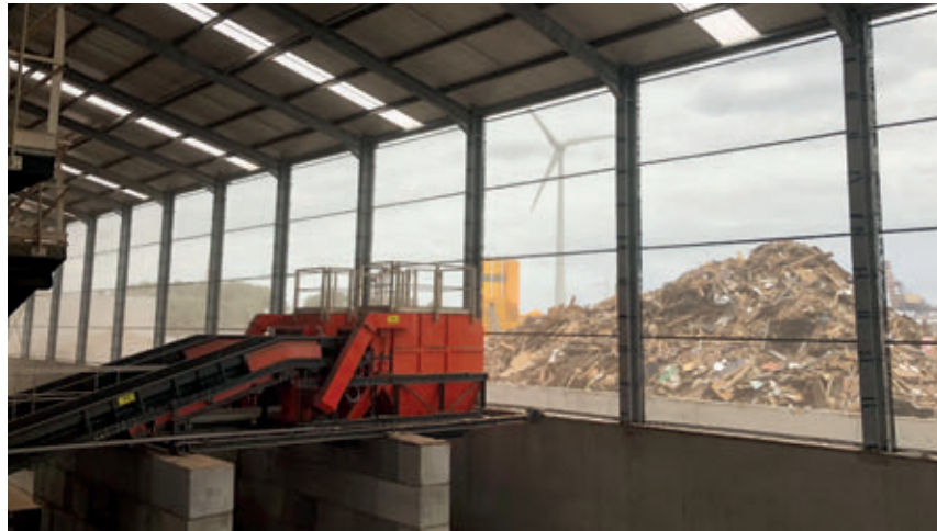
Technical textiles offer a uniform or architectural exterior while providing transparency from inside, supporting an optimal indoor climate with sufficient light, air, and ventilation.
