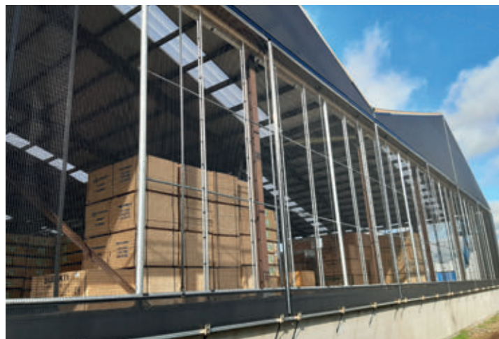
Adjustable side panels offer flexible open and closed configurations, ensuring that stored goods remain protected from the elements whilst maintaining ventilation.
