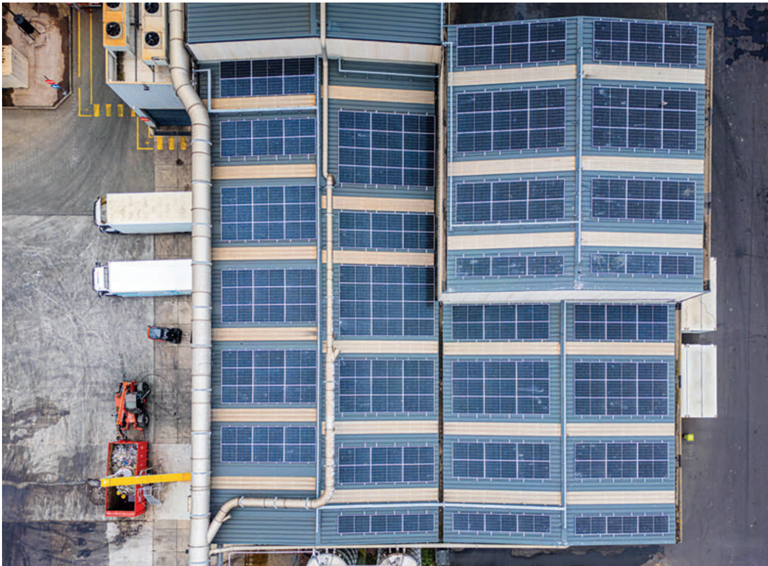
Darling Ingredients consistently invests in its facilities to optimise its production processes and reduce energy and water usage, as exemplified by Sonac's solar panel park in North Sea Port.
