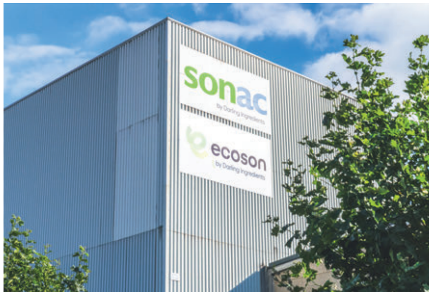
Darling Ingredients' North Sea Port facility is also home to Ecoson Recycling, which collects organic waste streams from the food and catering industry and transforms them into green energy.
