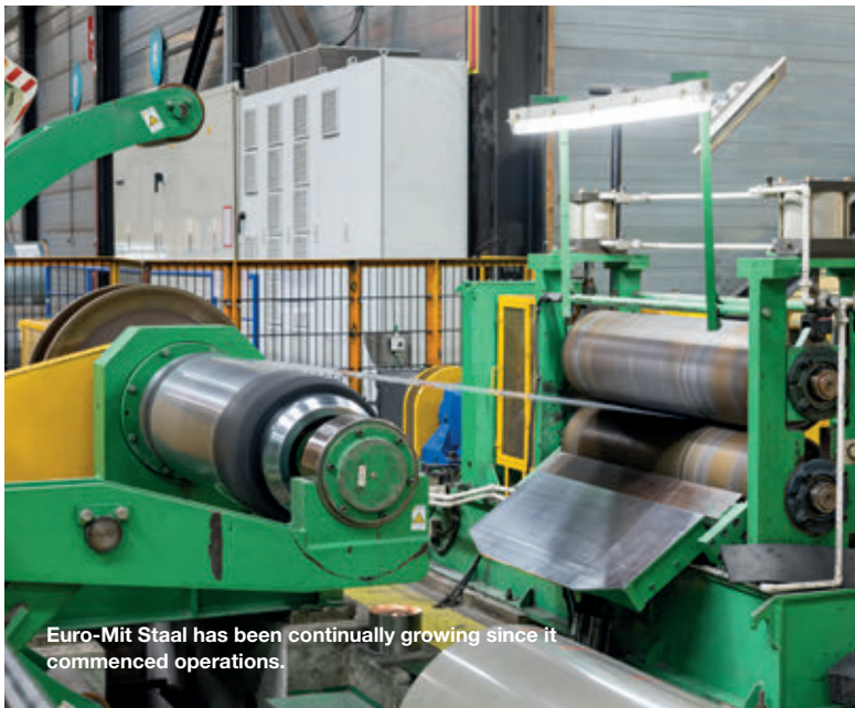
The installation of the new machine has been a complex, technical challenge.
