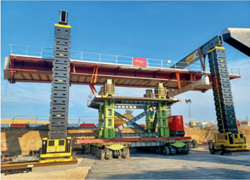
Much more than just a crane rental company, Aertssen Lifting conducts complex lifting and transportation operations, using telescopic and crawler cranes, jack-up and skidding systems, and SPMT transport equipment.
